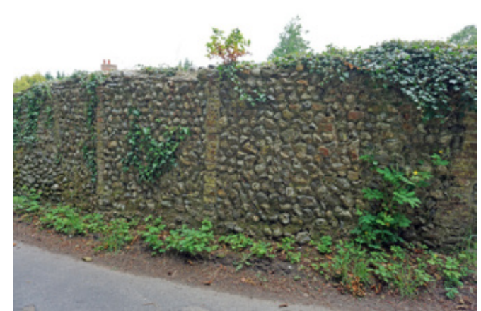
Section of red brick and flint wall fronting the graveyard of Stody Church shown with patches of vegetation growth
