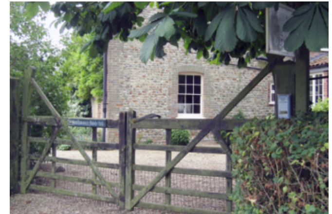
Rear elevation of Stody Hall with wooden gate
