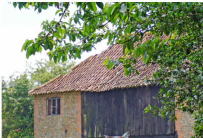
Roof in need of repair
