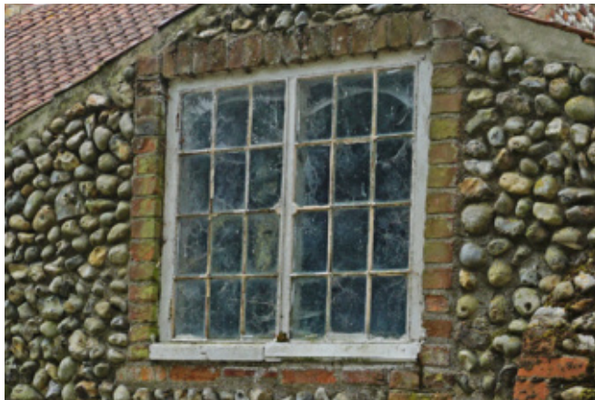
Window in need of maintenance
