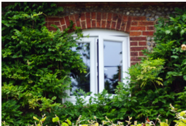
Inappropriate uPVC windows
