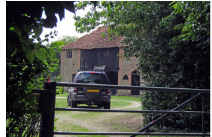
View of one of the grade II listed barns at Kendles Farm
