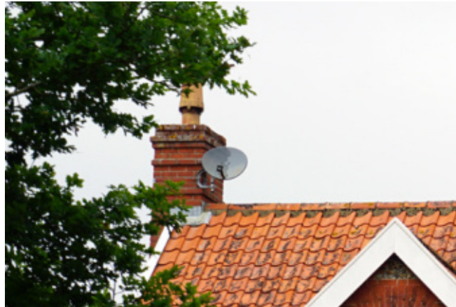
Visible satellite dish
