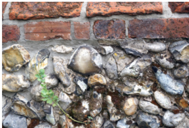
Cement pointing to an historic wall
